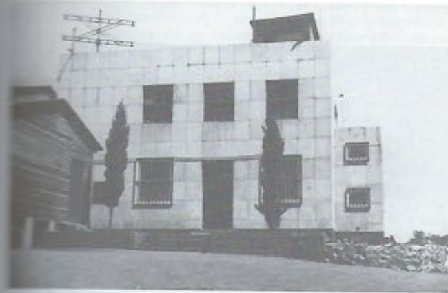
Figure 25. The BPI building (ca. 1940) in its wartime role as the headquarters of the Special Signals Section (subsequently Special Signals Services), South African Corps of Signals, with some of the wooden-framed RDF antennas mounted on the roof. (Reproduced by kind permission of Dr Mary Davidson.)
