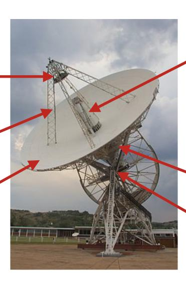
Feed housing (feed horns receivers and support structure)
