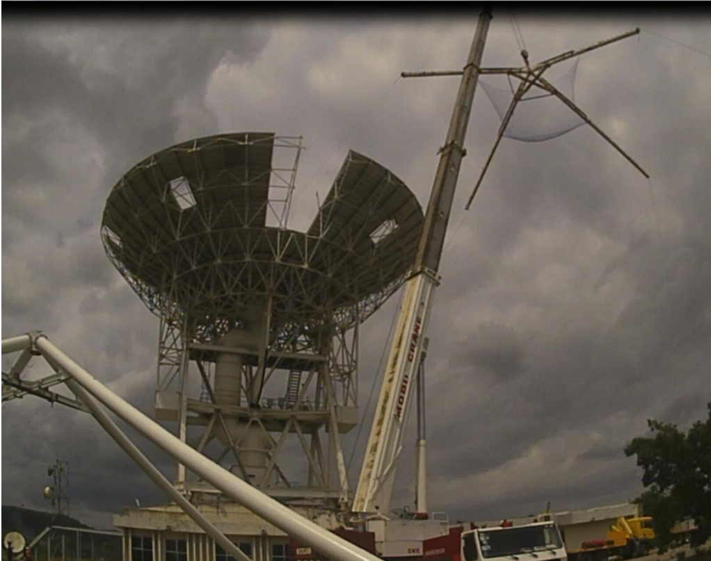
Quad legs - installation
