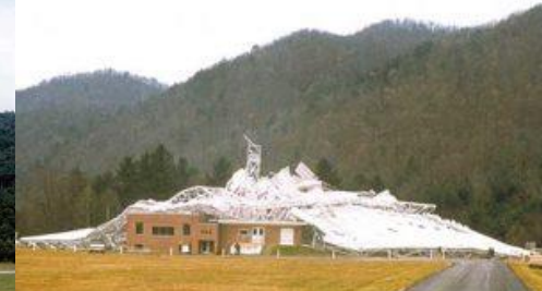
300 ft telescope, Green Bank – collapsed!
